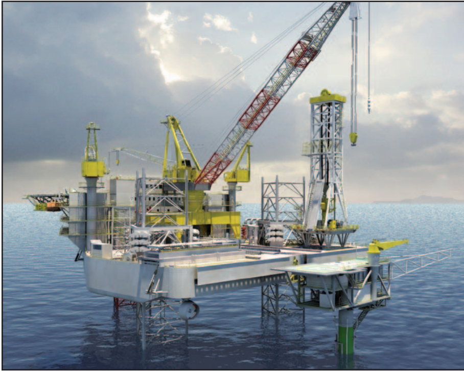
Power for the diesel-electric propulsion, as well as the working and hotel loads, is provided by four GE Transportation diesels — one eight-cylinder V228 and three 16-cylinder engines.
